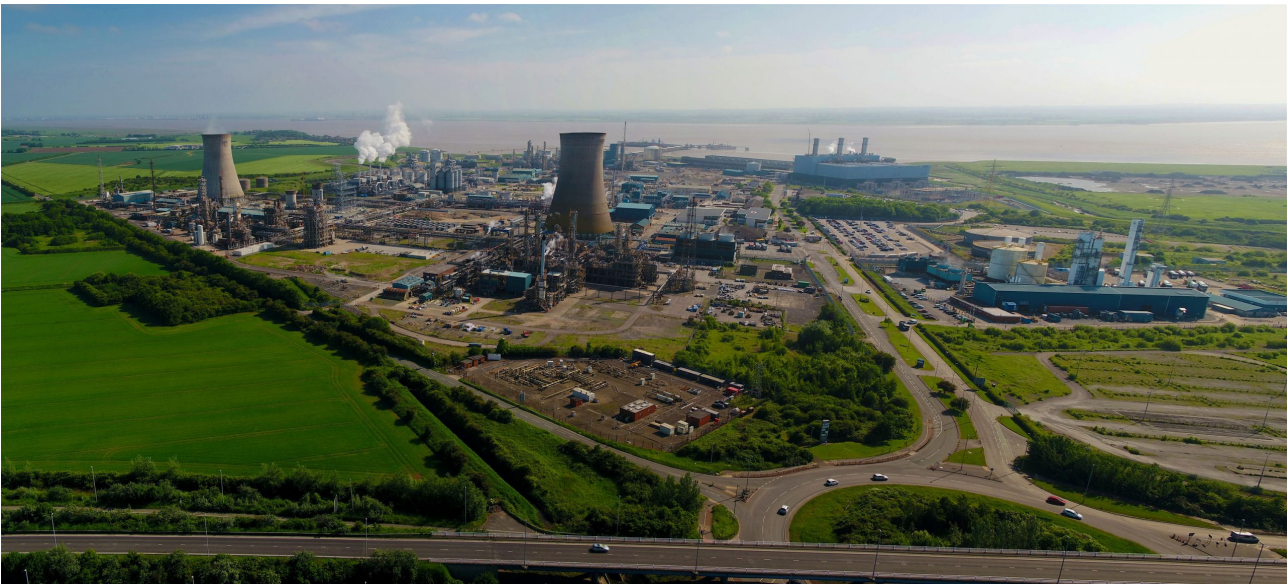
Photo of Saltend Chemicals Park (credit: px Group)
